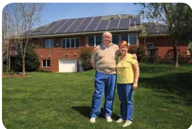
David and Jan Barrow's 16.9 kW solar PV System
